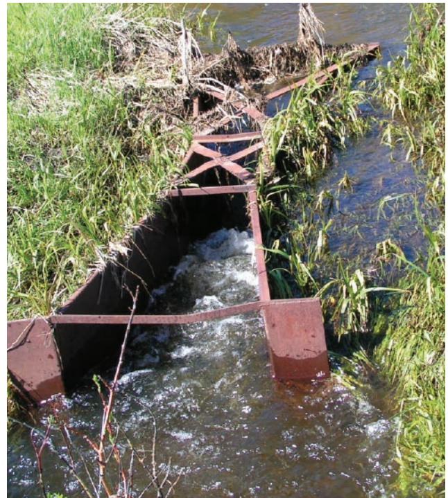
This flume is not functioning properly. It is choked with vegetation, out of level, and too small to capture the entirety of diverted flow.
